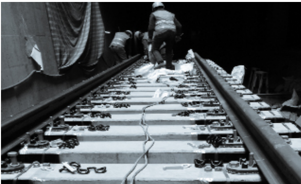
Installation of Sleeper Boots
