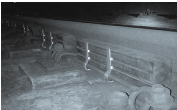
Installed Rail Dampers
