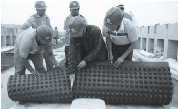
Installation of Track Mats
